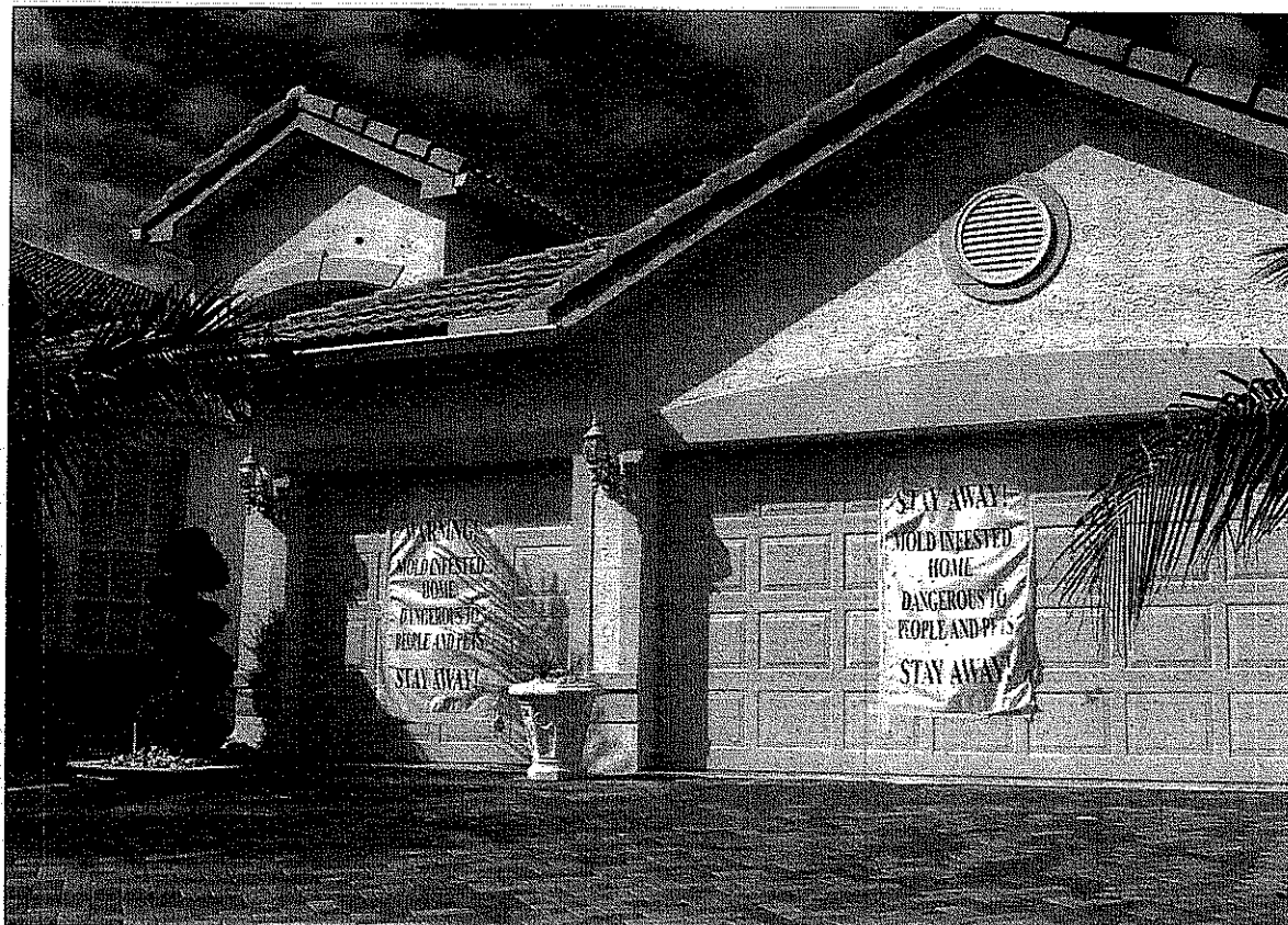
Shirlee Daily's home at 19216 Skyridge Circle with signs posted warning of mold. She claims she was forced out of her home because of toxic mold.
